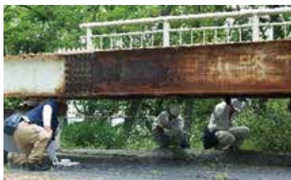
Inspecting a Steel Bridge
