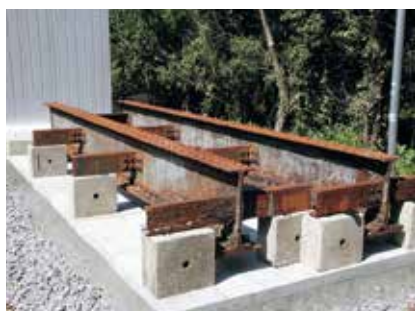
Steel rivet girder
