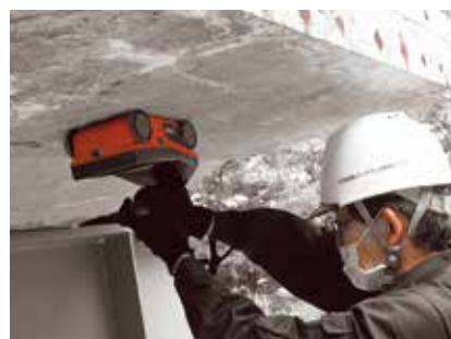
Non-destructive inspection by electromagnetic wave radar
