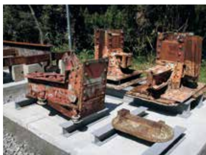
Steel truss bridge and supports
