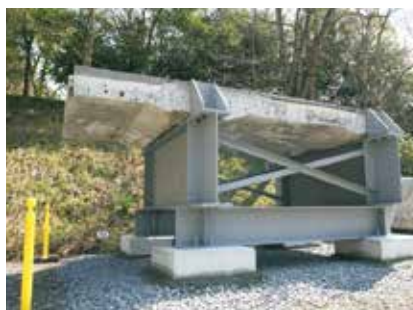
Reinforced concrete slab
