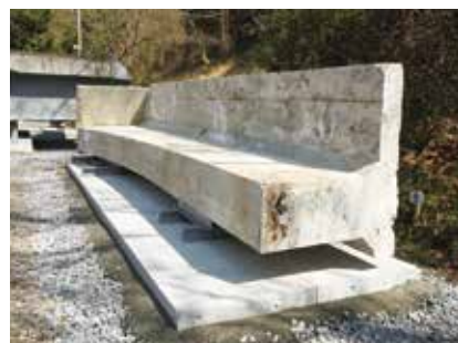
Reinforced concrete girder
