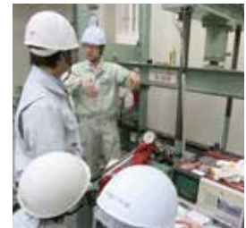
Loading of steel structure
