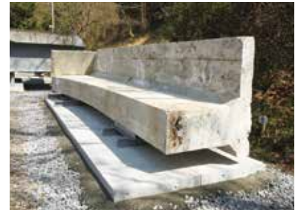
Reinforced concrete girder
