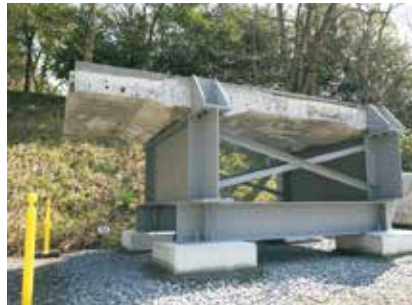
Reinforced concrete slab
