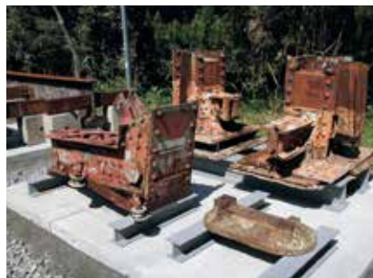
Steel truss bridge and supports
