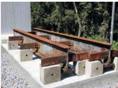
Steel rivet girder
