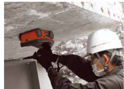
Non-destructive inspection by electromagnetic wave radar
