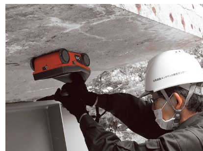
Non-destructive inspection by electromagnetic wave radar
