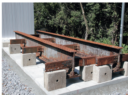
Steel rivet girder
