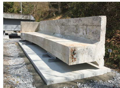
Reinforced concrete girder
