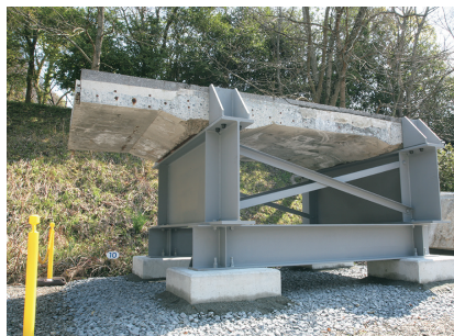
Reinforced concrete slab
