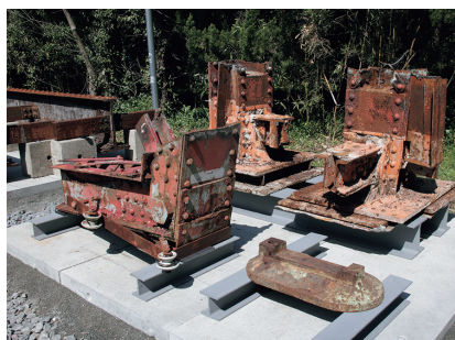
Steel truss bridge and supports
