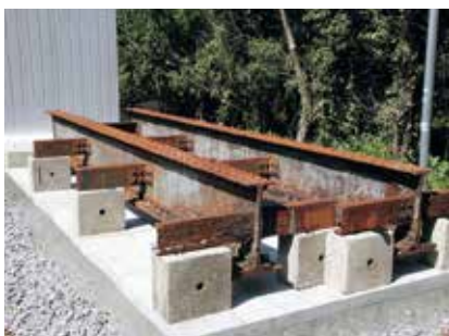
Steel rivet girder
